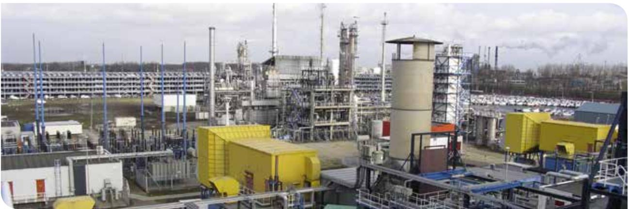
— A CO-generator consists of a desalination plant and a boiler. Smallest organic impurities result in production of carbonic acid, which increases the risk of corrosion considerably. It is important to detect impurities quickly and reliably.
